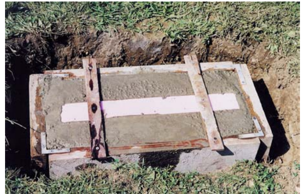
On the right, the poured base with setting form in place
