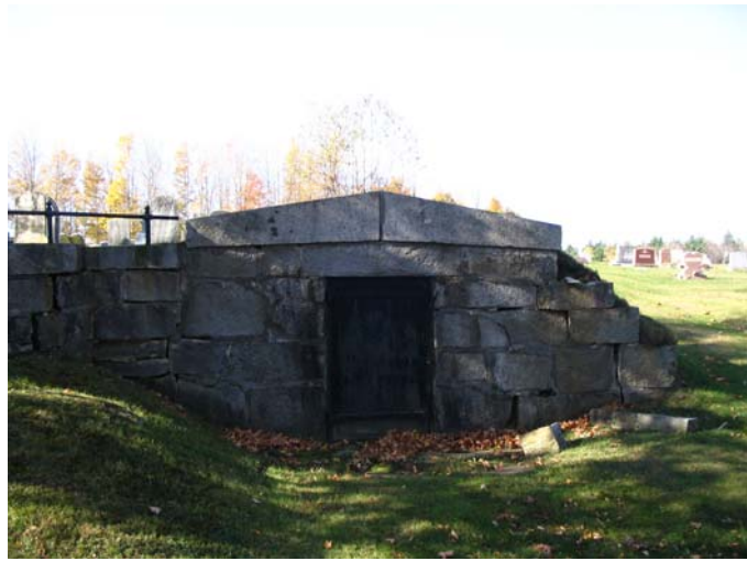
Figure 16. Preliminary recommendations include stabilizing the tomb structure by rebuilding the façade and installing an improved drainage system.
