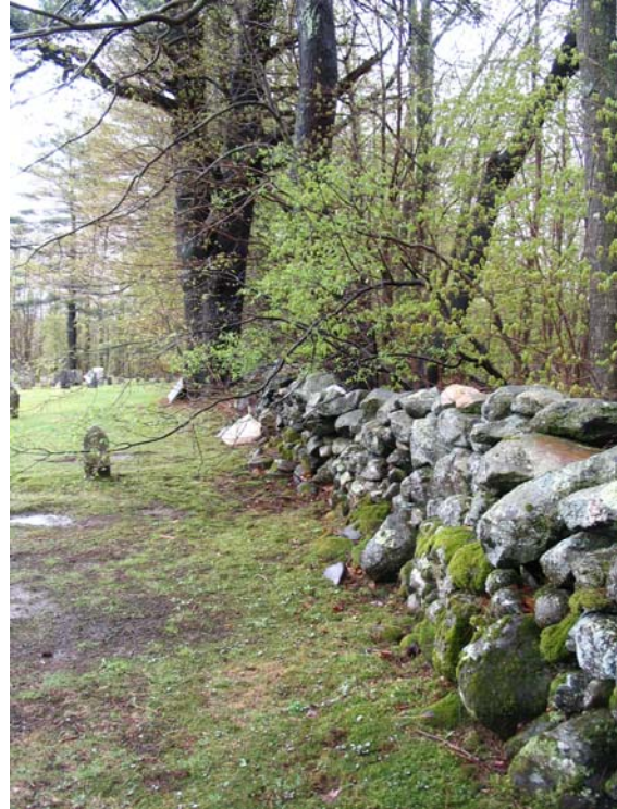
Figure 14. The dry-laid stone wall along the cemetery's south edge may be one of its oldest remaining original features.
