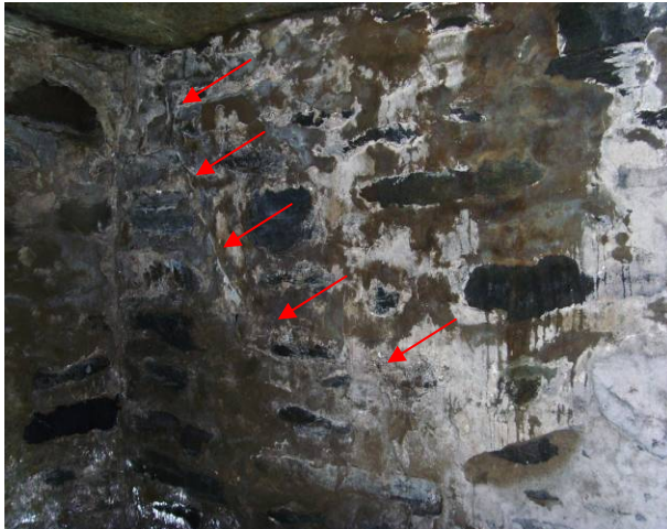
North Wall of Tomb Interior (Arrows show cracking pattern)
