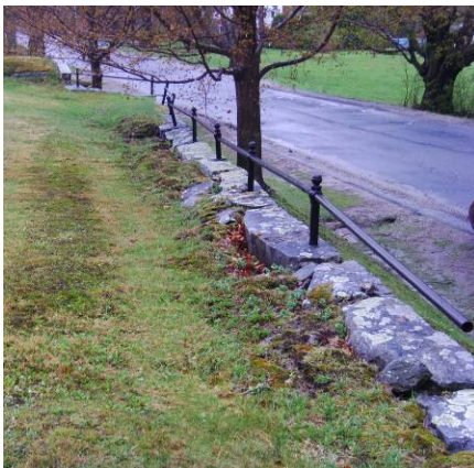
Sinkholes behind Wall
